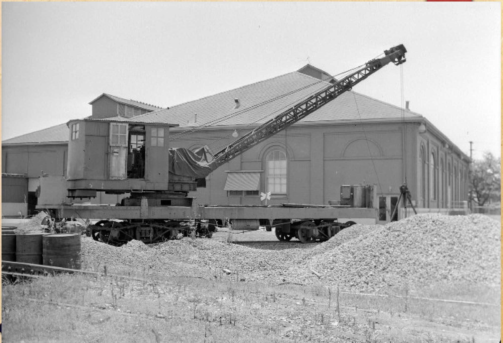
NOPSI "hoist car" at Napoleon Yard
